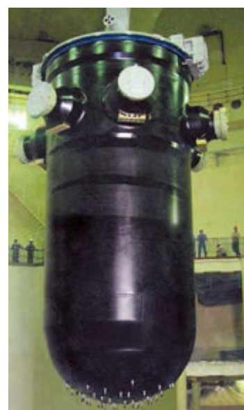
Installation of reactor vessel
