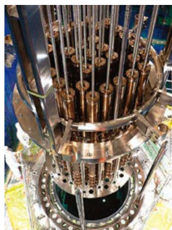
Installation of Core internal
