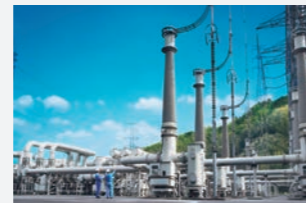
550kV gas insulated switchgear
