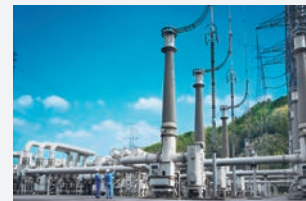
550kV gas insulated switchgear
