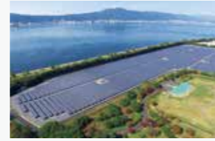
Photovoltaic power generation system (Shiga, Yabasekihantou mega solar power plant)
