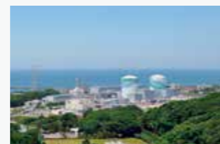
Nuclear power plant (Sendai Nuclear Power Station)
